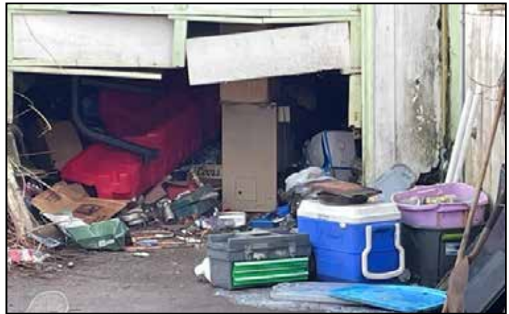
The City of Sheridan rental house at the corner of Mill and Morgan has been allowed to remain in this condition for the past few years. New City Manager Heidi Bell (who inherited this issue) said she will make this situation one of her priorities.
