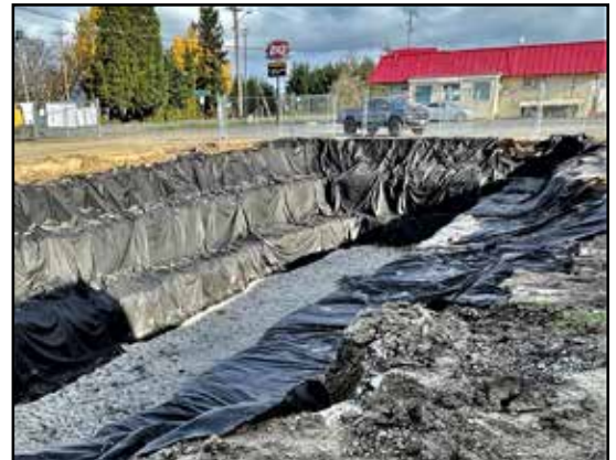
This giant hole will be filled with two fuel tanks.
