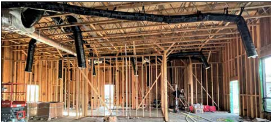
Construction of the new 5,000 sq. ft. Valley Market is well underway.
