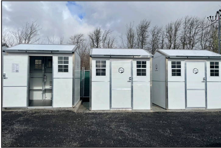
Frontal view of three Pallet Shelters.
