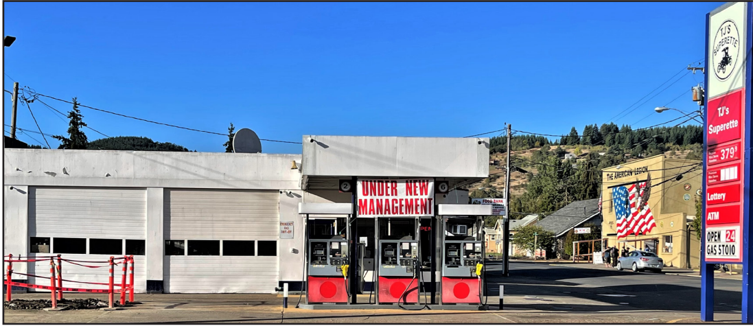
TJ's Gas Station, 107 W. Main in Sheridan, on Saturday, Oct. 2, prior to its demolition.
