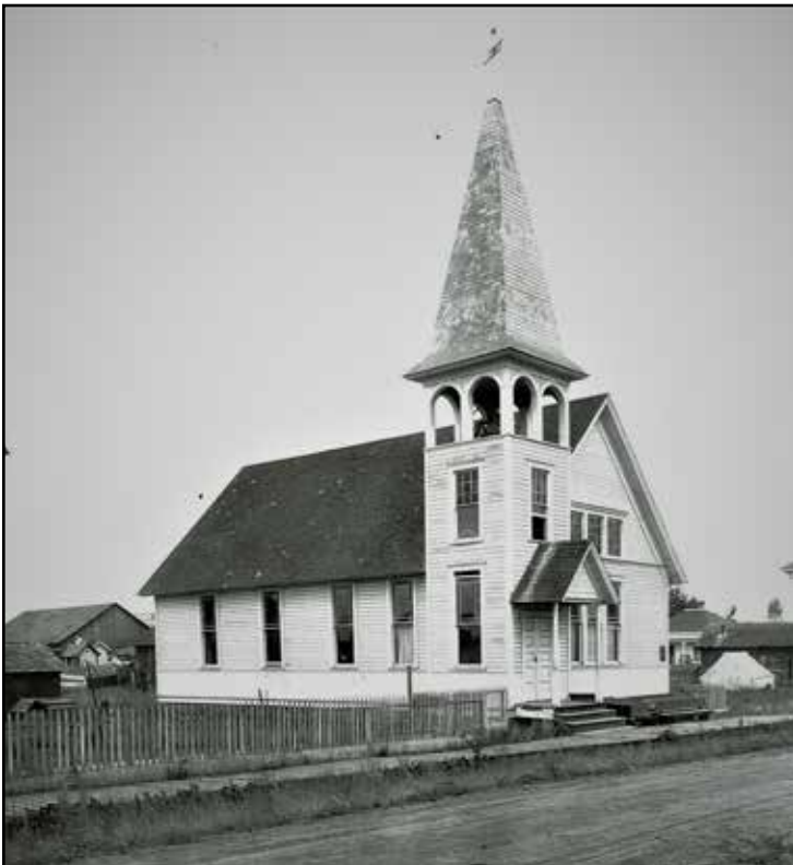
The Congregational Church was built in 1892/93 at 220 SW Monroe Street. It later served as the Mennonite Church for several years. The Assembly of God congregation was the next owner, until they sold to the Sheridan Baptist Church. Dick Jordan purchased the old church in 1996 and converted it into a four bedroom house. The original siding and bell tower remains, but the tall steeple has been removed.
