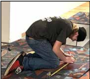
Volunteer Isaac, 13, measured and cut carpet for a new ramp inside.
