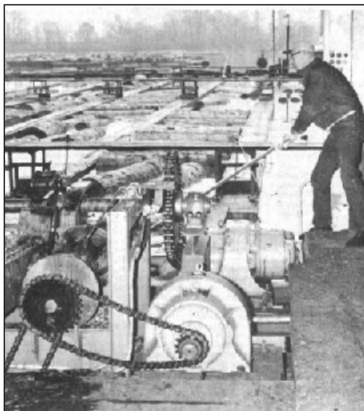
New automated equipment now lifts logs from the US Plywood Company pond to begin the journey through the new and automated lathe as the mill gets back into production after a long closure and installation of new machinery. A US Plywood employee performs, one of the few non-automated jobs left, guiding a log into position, so it can be lifted from the water.
