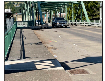
The new bridge railing on South Bridge Street.
