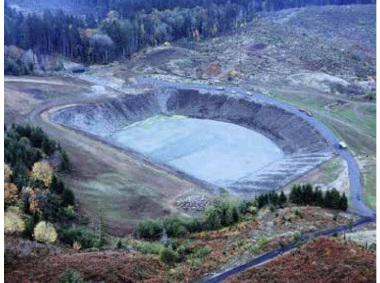
Construction of the Stoney Mountain Reservoir, located about nine miles north of Sheridan, was completed in 2009.
