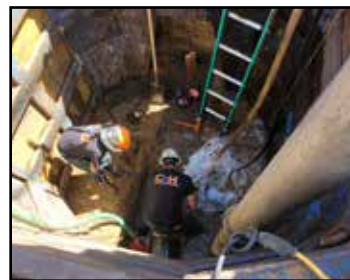
Workers repair a leak that developed on the main water line for SW Sheridan area.
