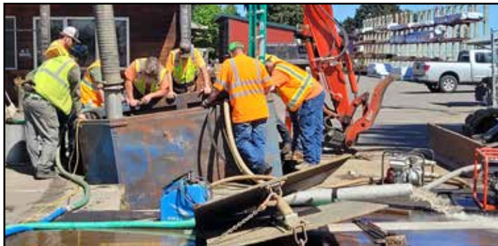
Sheridan Public Works keep an eye on the workers making a pipe repair on a main water line leak at the intersection of S. Bridge and SW Railroad St.
