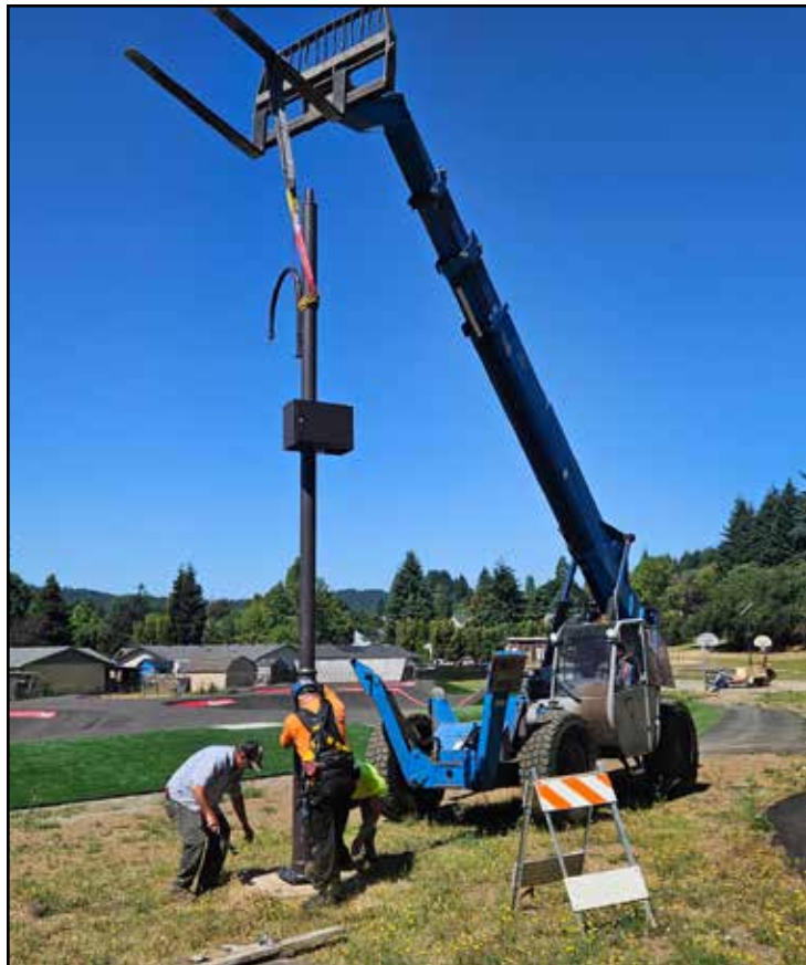
Last Tuesday, the City of Willamina received assistance from Stuck Electric and the Hampton Lumber Twin Maintenance Crew, who installed two solar light posts at Oaken Hills Park in Willamina.
