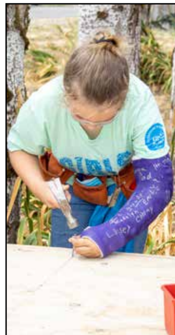
Cassidy did not let a broken arm slow her down as she concentrated on nailing down the plywood in the Girls Build Ramp Project.
