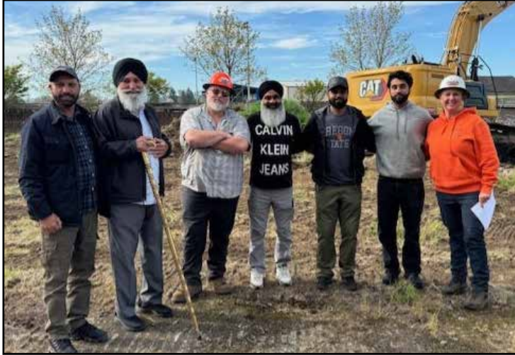
Partners Erick and Melissa Poland (orange hat and hoodie), Gurdeep Dhalial (second from left), and Paul Johal (middle), along with family members, prepare to break ground for a new apartment complex in Sheridan. All partners have local ties to the area.
