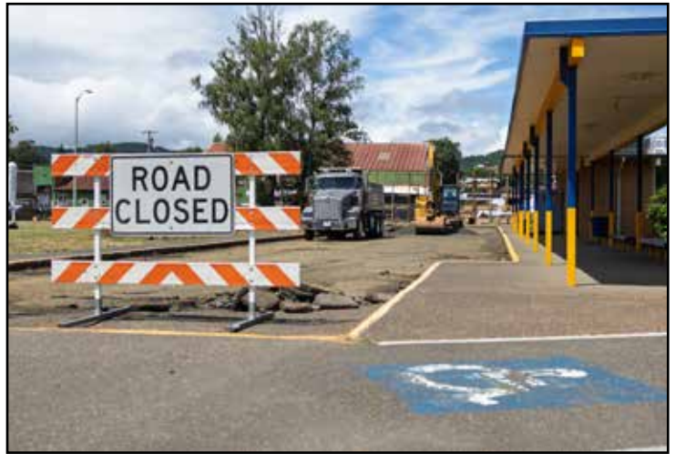
Construction crews began work on the Sheridan High School bus pickup area and parking lot immediately after Sheridan Hometown Days. The project is one of many improvements being funded through the school bond approved by voters last year.
